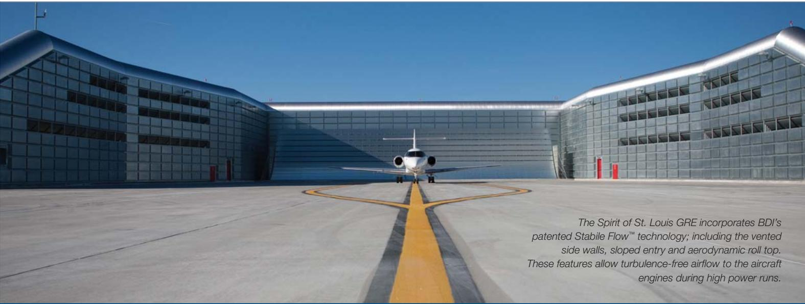
*The Spirit of St. Louis GRE incorporates BDI's patented Stable Flow™ technology; including the vented side walls, sloped entry and aerodynamic roll top. These features allow turbulence-free airflow to the aircraft engines during high power runs.*
