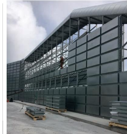
Installing special acoustic panels that block aircraft engine noise and prevent acoustic reflection. (PortsToronto)
