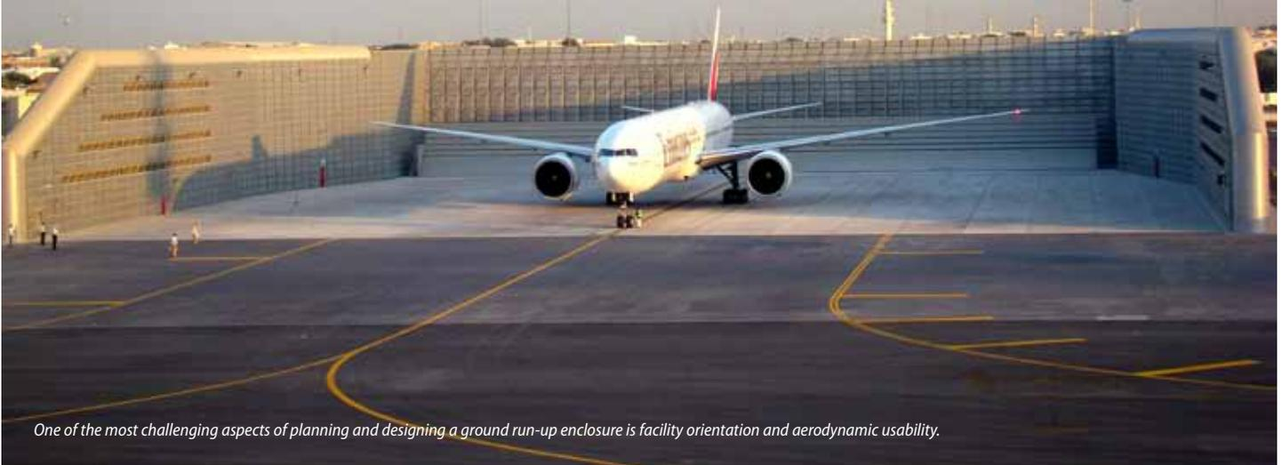
One of the most challenging aspects of planning and designing a ground run-up enclosure is facility orientation and aerodynamic usability.
