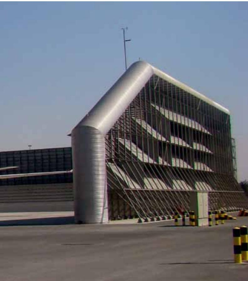
facility and inside the GRE. Instruments recorded noise levels during both the open-air and in-facility engine run-ups. "The difference in noise levels between the open-air and in-facility engine run-ups is called insertion loss" explains Bergin. After run-ups were performed with two aircraft, a Boeing 777-300ER and an Airbus 340-500, the necessary data was recorded to determine the insertion loss each aircraft.
