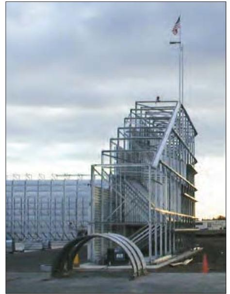
**The framing seen here will be covered with a pre-engineered metal skin. The Garrison Company worked with Butler Manufacturing to design the custom girts seen in this photograph.**
