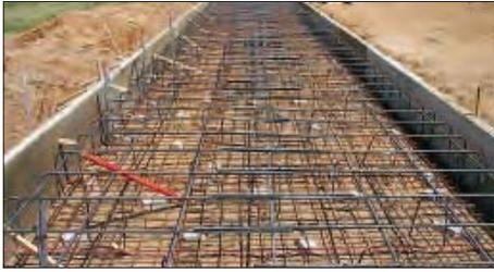
**The large vertical walls subject the structure to strong wind loads, while lightweight construction results in relatively low structural loads. A specialized foundation meets the support needs of the structure without adding more rigidity than needed.**
