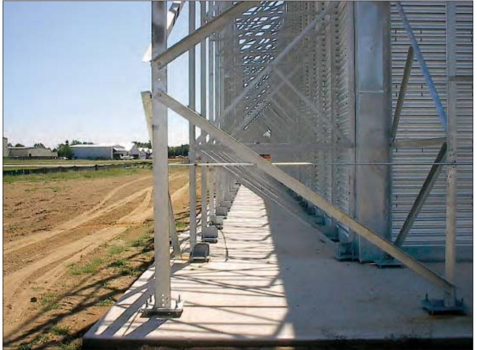
**The GRE frame features extensive cross bracing to provide sufficient wind resistance relative to the height of the structure.**
