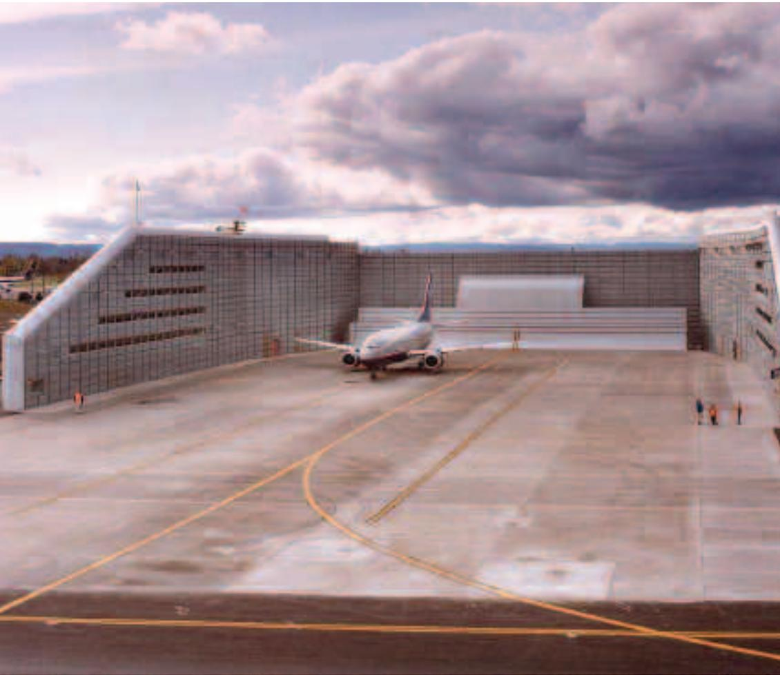
PDX and TPA utilize a new Stable-Flow™ Ground Run-up Enclosure design for noise abatement.
