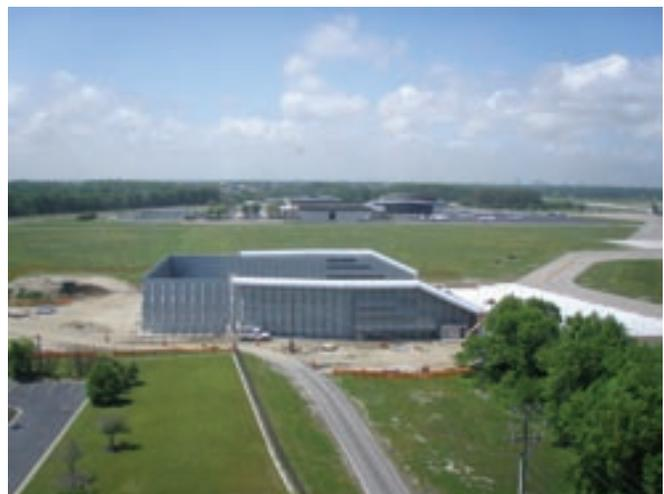
tenants and transient aircraft. New airport regulations developed by the Airport Authority require all engine runs above 50% power be performed in the GRE provided the aircraft can fit in the facility, which can accommodate up to a B737-800. ■
